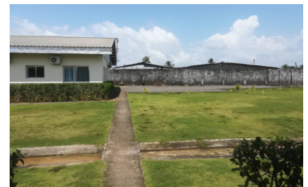
Site of the proposed school building.
